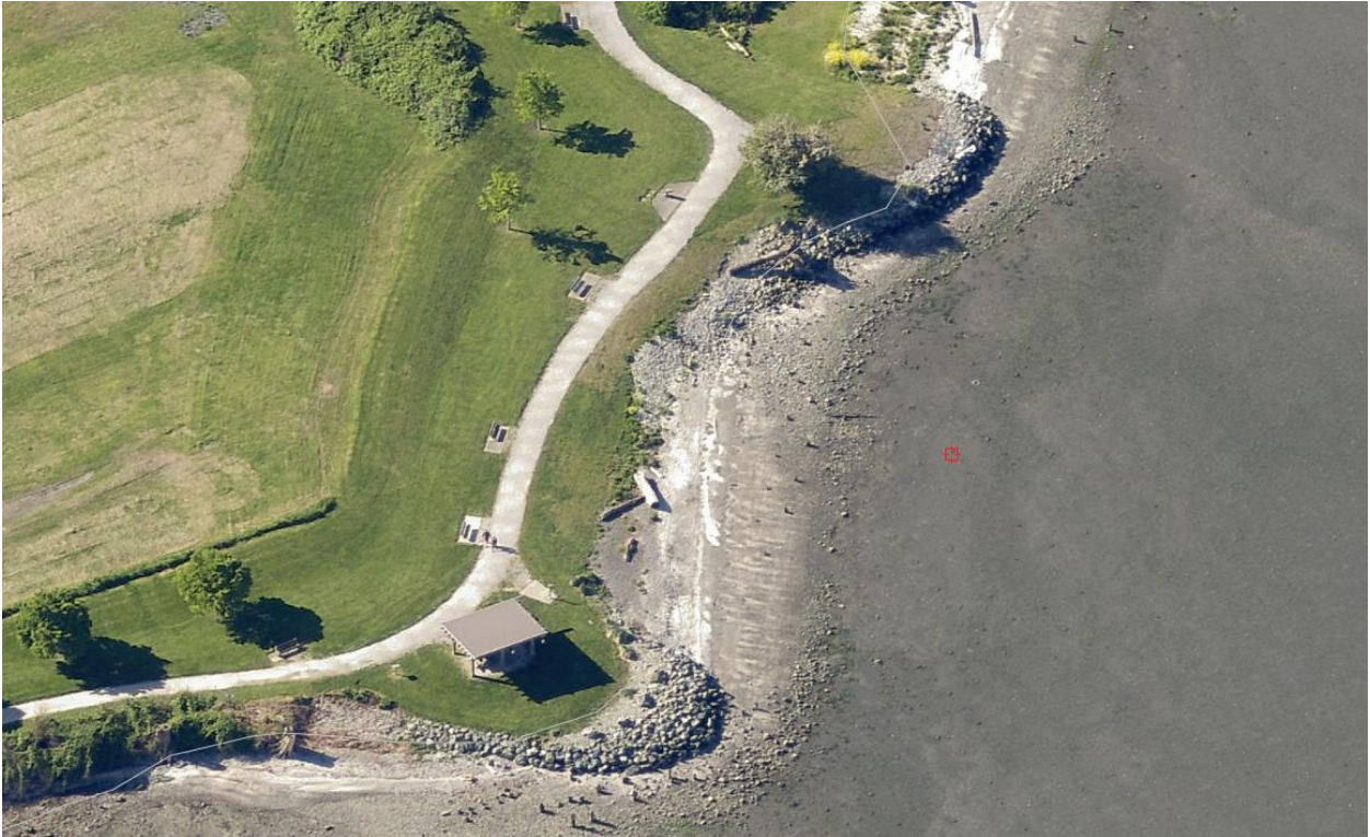
Figure 1: Phase 1 completed shoreline restoration improvements, Marine Park
