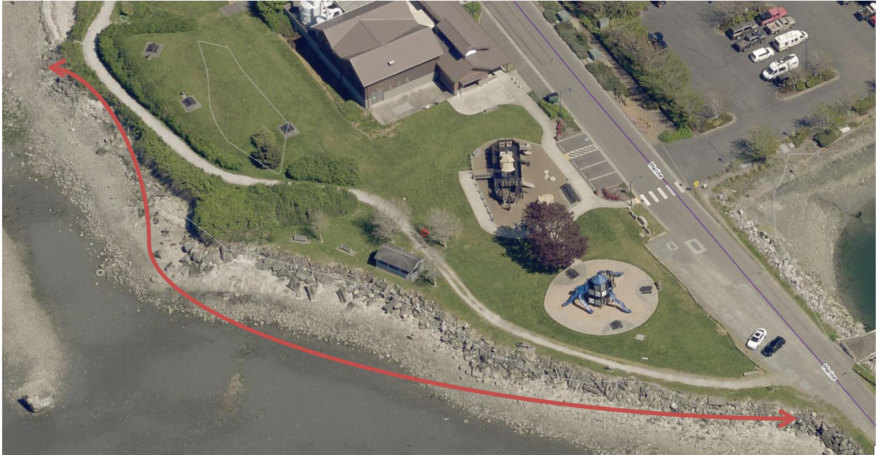
Figure 3: Aerial Photograph of Project Site, May 8, 2020
